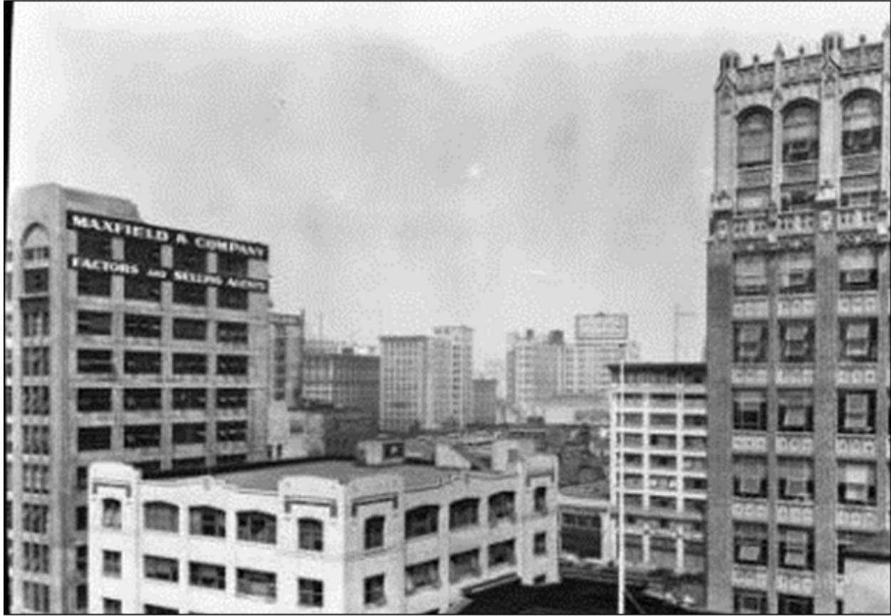
Figure 4. Maxfield Building (left), note painted signage reading “MAXFIELD & COMPANY FACTORS AND SELLING AGENTS” (USC Libraries Special Collections, 1927)
